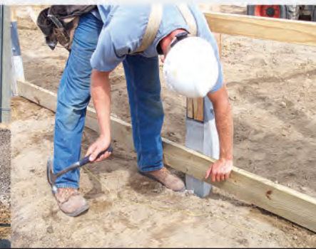
ATTACH SPLASH BOARD
